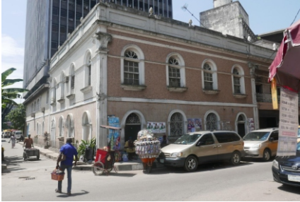
Water House © Mark Raymond
