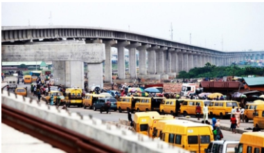
LAGOS LIGHT RAIL PROJECT BY CCECC
