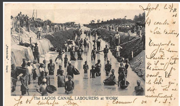
Construction of Lagos Canal. Possibly the Macgregor canal was built between 1903 and 1904 during the colonial administration of William Macgregor. Circa: 1900's
